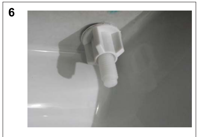
Once the seat and pan match, fully tighten the nut.
