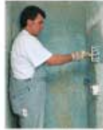
1. Priming: Prime absorptive mineral gypsum-based substrates and plaster boards with Primer G.
