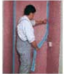
3. Fit the PCI-waterproofing Pecitape with PCI-Lastogum X in corner joints and floor/wall junctions.
