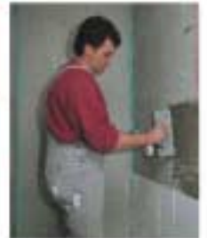
6. After the waterproofing PCI Lastogum X is dry tiles can be laid with PCI-Tilefast 6 Flex or Rapidflex.
