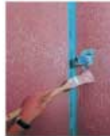
4. Place PCI-waterproofing gasket (wall) over the pipe connection protruding from the wall and cover with PCI-Lastogum X.
