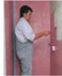
2. Apply undiluted PCI-Lastogum X to the substrate as a first protective coating to cover its entire surface.
