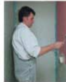
5. After an evaporation time of 2-3 hours apply the second protective coating with PCI-Lastogum X.
